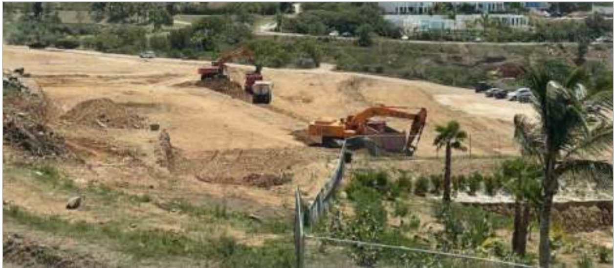
Plate 3-3 Mass earthwork process, including clearing the land with excavators, moving soil, and compacting the ground to ensure a stable foundation for construction.
