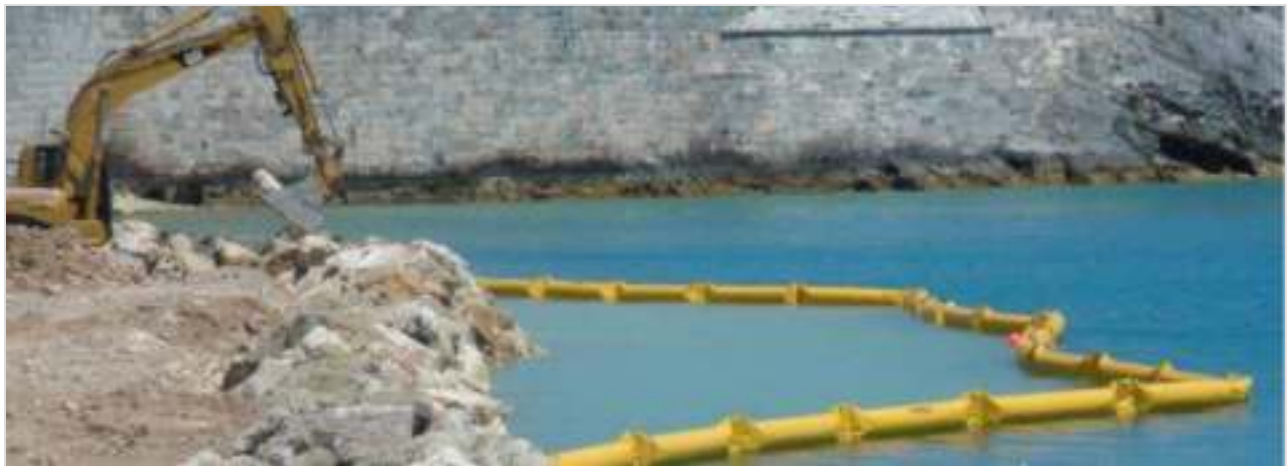
Plate 3-6 Example of a turbidity barrier
