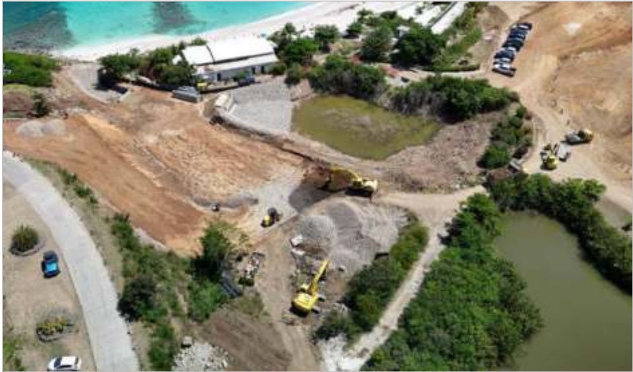
Plate 3-5 Example of storm detention ponds with outflow drainpipes at head wall and riprap protection.
