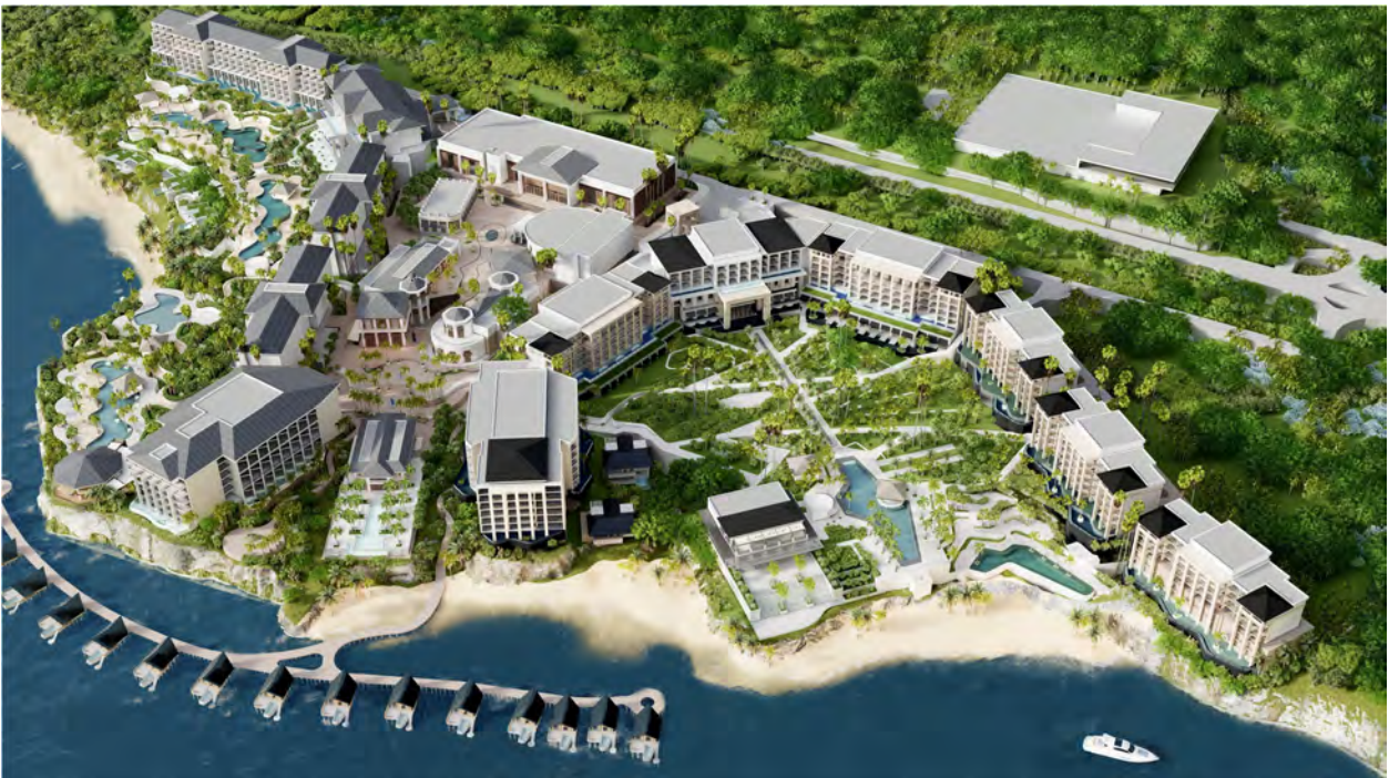
Figure 4-2 Render of Phase 2 expansion looking to the southeast (TRS in the foreground and GP in the background)
