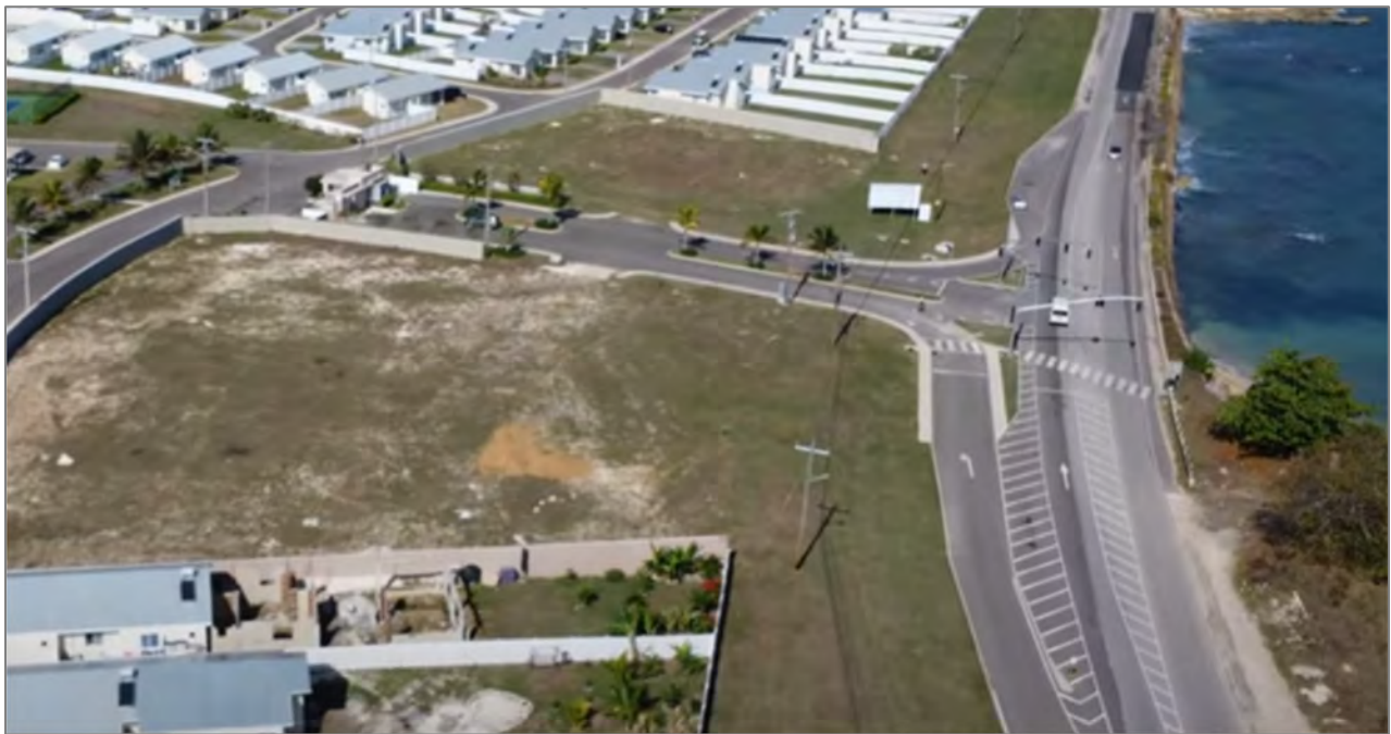
Plate 5-27 Aerial view of the Oceanpointe intersection
